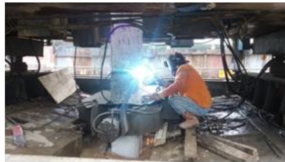
Figure 7. Pile Welding Source: Documentation, 2023
