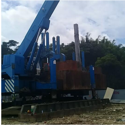
Figure 2. Hydraulic Jack In Pile Source: Documentation, 2023
