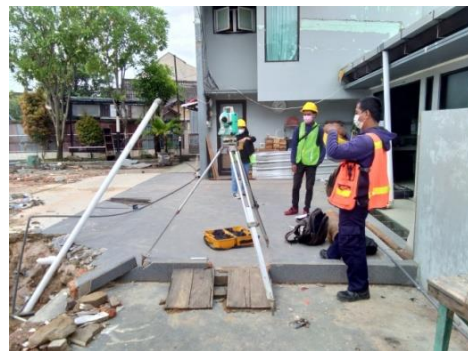
Figure 5. Measurement and Determination of Pile Points using Theodolite Source: Documentation, 2023
