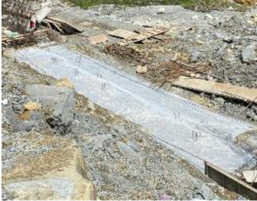
Figure 7 The Installed Mini Pile Foundation Viewed From Above Source : Documentation, 2023
