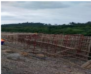
Figure 11 Formwork Installation Work Source : Documentation, 2023
