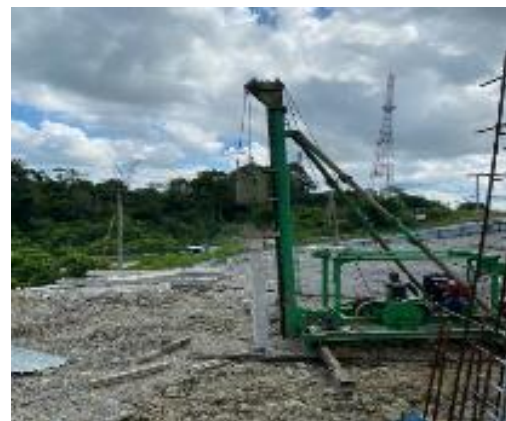
Figure 6 Installation of Mini Pile Foundations Using a Drop Hammer Tool
