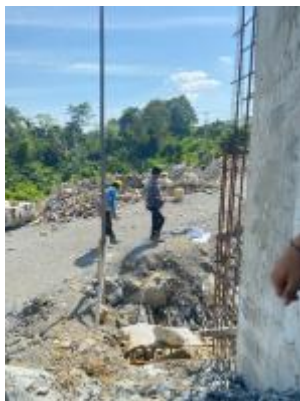
Figure 4 Work of Installing Iron Stakes After Receiving Pile Point Locations
