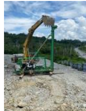
Figure 5 Preparation of the Drop Hammer Equipment at the Pile Points Where Iron Stakes Have Been Installed
