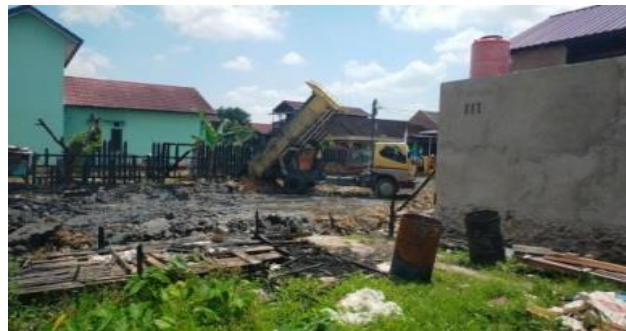
Figure 5. Heap of Excavated Land
