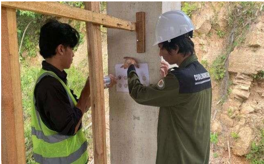
Figure 4.1 Column Hammer Test Self-Documentation in the Field
