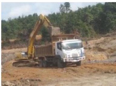
Figure 4. 3 Preparing the Work Area (Source: Personal Documents, 2023)
