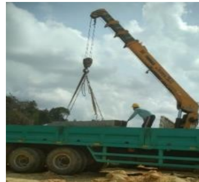
Figure 4. 15 Material Mobilization (Source: Personal Documents, 2023)
