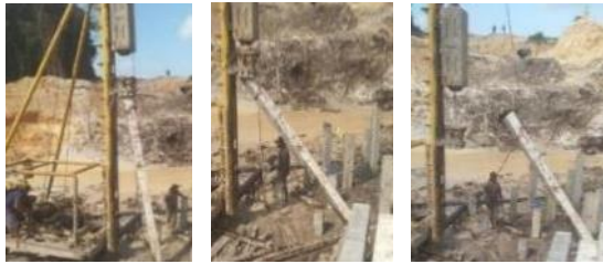
Figure 4. 6 Pole lifting
