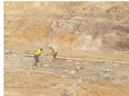
Figure 4. 12 Pole Cutting (Source: Personal Documents, 2023)
