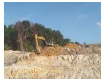
Figure 4. 2 Work Area Cleaning (Source: Personal Documents, 2023)
