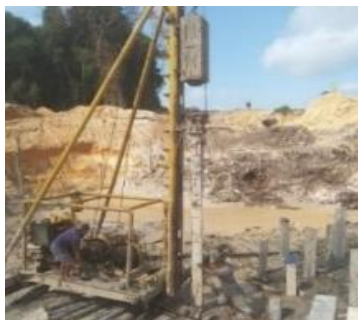
Figure 4. 7 Upright Control of Piles
