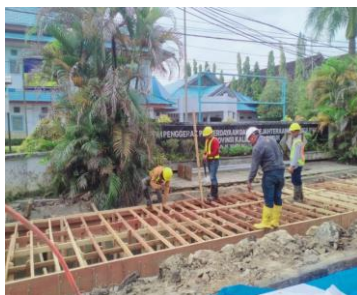
Picture 3. Formwork (Source : Personal documentation, 2023)
