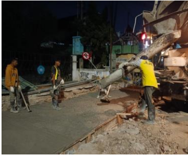
Picture 5. Concreting Work (Source : Personal documentation, 2023)
