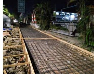
Picture 4. Reinforcement Work (Source : Personal documentation, 2023)
